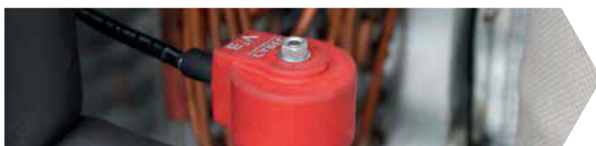
Electronic expansion valve
